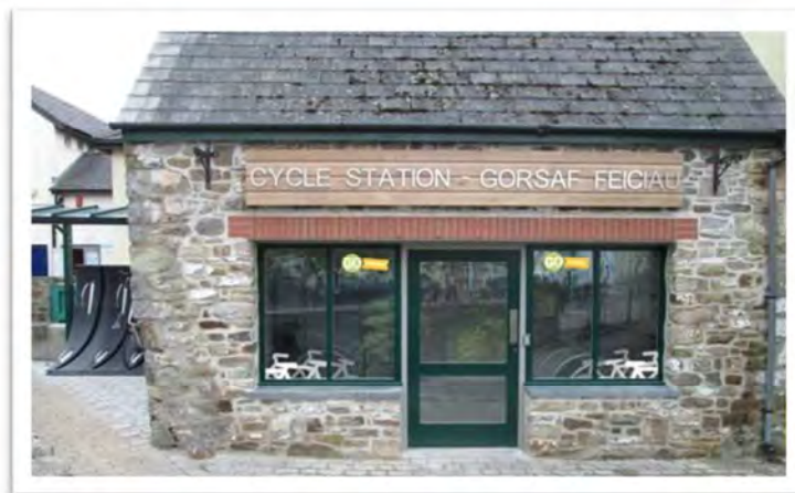
Photo Above; Haverfordwest Cycle Station
