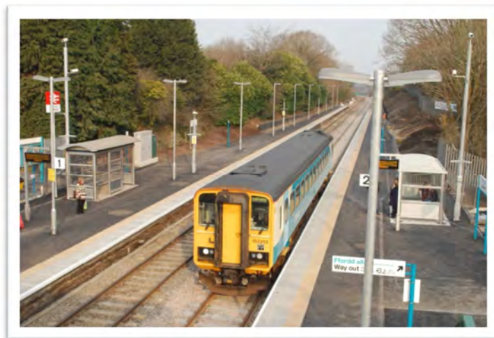
Photo above; Redeveloped station at Gowerton.
