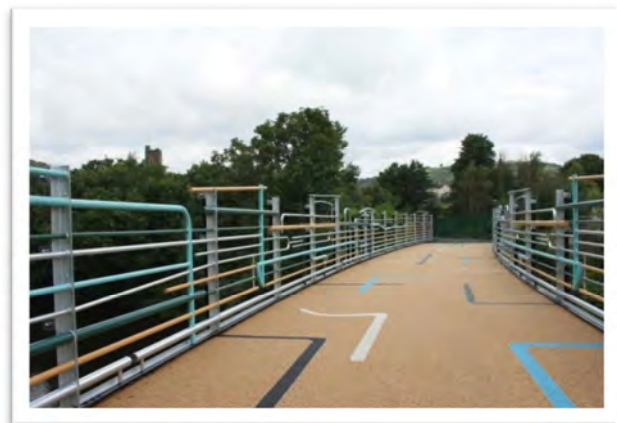
Photo above: Clydach Connect 2 Bridge
