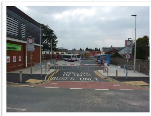
Photo above: Improvements to rural interchanges – Ammanford Bus station
